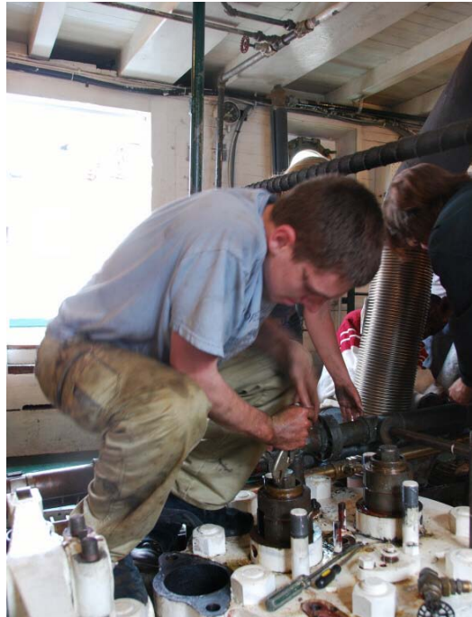
Grant removes a valve cage using vice grips
